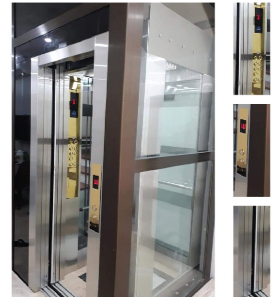
Cab 30 - inox, kính quan sát (tempered glass) Trần trang trí (car ceiling): CS - 30
